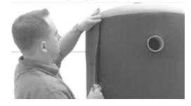
6. Stick second adhesive tape over the butt joint of the insulating jacket.
