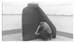
5. Fasten the start and end of the insulating jacket at the adhesive tape applied in 1.
