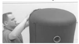
9. Seal the butt joint with additional insulating tape.
